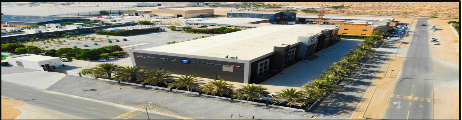
A2C Services LLC, Al Jazeera, Ras Al Khaimah - UAE
